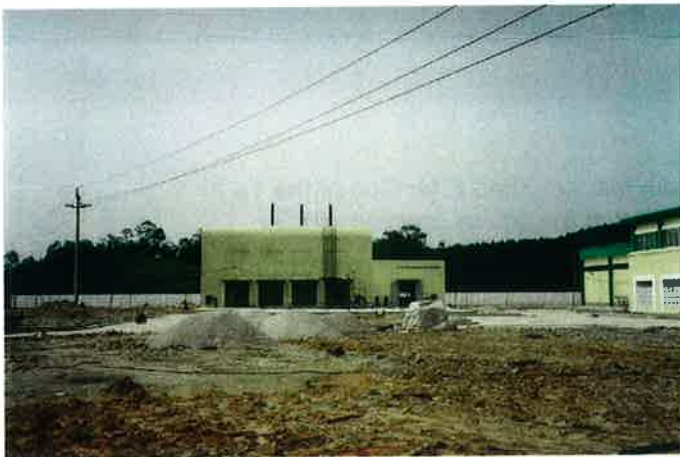
SGJ factory in the early days of construction
